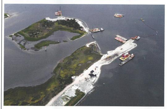
Mile Point scheme one of the first breakwater construction projects ever to use Trimble Marine Construction (TMC) software and Teledyne BlueView sonar to collect motion-compensated 3D point clouds and create a 3D model from the moving barge platform in real-time
