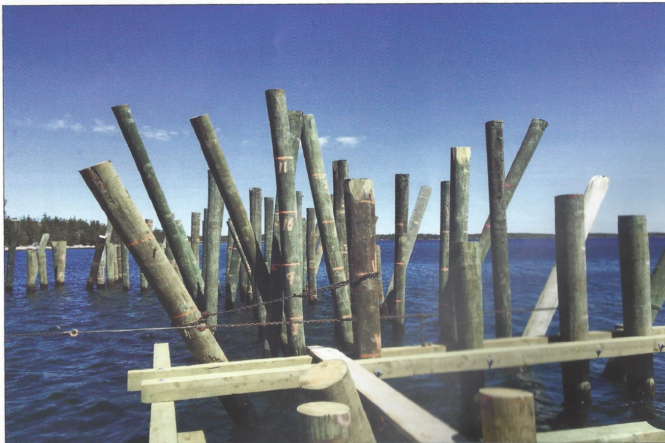
Above, the crew installed the equipment bracket high on the lead to protect the two GPS antennas and the pitch/roll from the free-swinging piles as they were positioned in the lead. Left, after the timber piles were placed, they were cut off to design elevation and the wooden cribbing installed in preparation for installation of the concrete cap. The batter piles provide extra strength to the structure by resisting heavy lateral or inclined loads.
