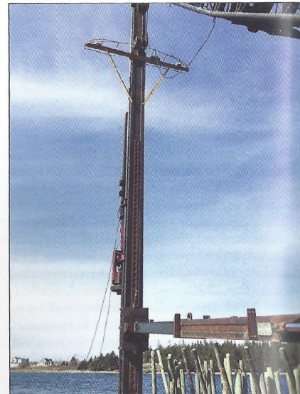
Above, the crew installed the equipment bracket high on the lead to protect the two GPS antennas and the pitch/roll from the free-swinging piles as they were positioned in the lead. Left, after the timber piles were placed, they were cut off to design elevation and the wooden cribbing installed in preparation for installation of the concrete cap. The batter piles provide extra strength to the structure by resisting heavy lateral or inclined loads.
